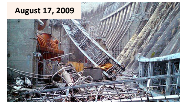
Destruction Sayano-Shushenskaya Hydroelectric Power Plant
