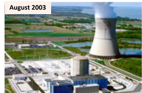
Davis-Besse Nuclear Power Plant
