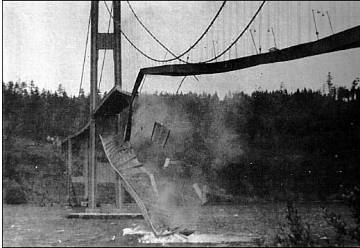
Figure 1 A 600-foot section of the Tacoma Narrows bridge crashes into Puget Sound as the bridge twists and torques itself to death. Mechanical engineers are warned early on that this can happen if they don't practice good engineering.
